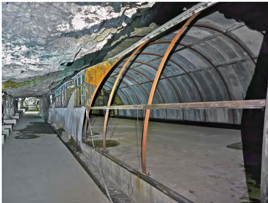
Fordham's Accommodation: Liddell Union gallery was enlarged here just sufficiently to house a parallel row of Nissen huts
